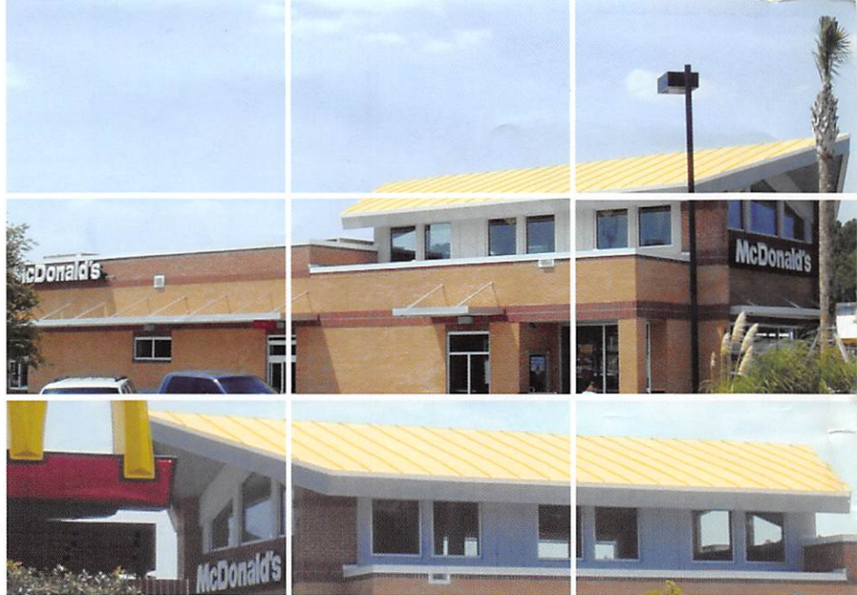
The Sarnafil Décor Roof System in custom yellow on top of McDonald's in Savannah, Georgia
